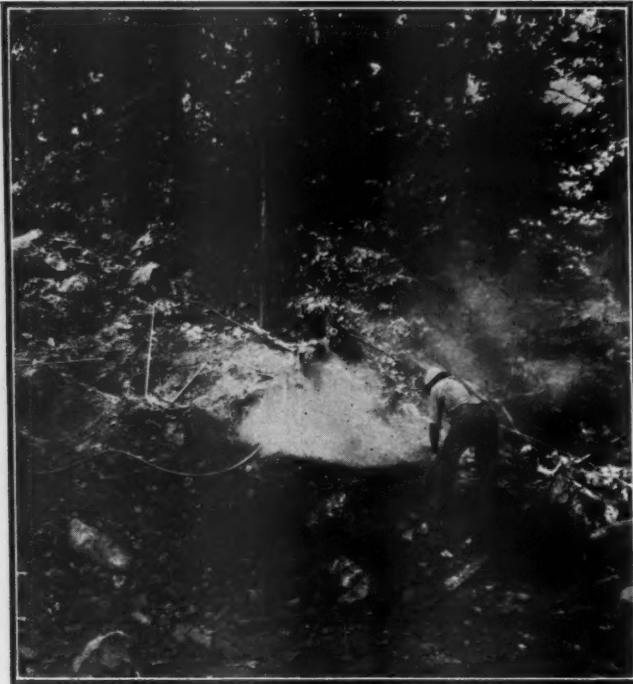
Air Drilling at One of the Pits
